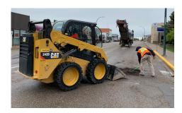
Overall, the project has given the Town a series of valuable outcomes. Milling from the removed asphalt will be repurposed to Coaldale's LINK Pathway Phase 1 construction. A small portion of the millings will also be used to create ramps at all intersections for easier pedestrian access.
